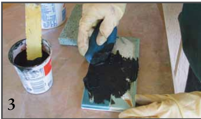
3 Apply grout to the tile surface with a flexible tool. Wear protective gloves.
