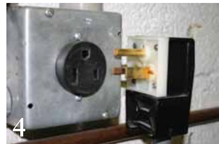
4 Unplug the kiln and inspect the prongs and insulation.
