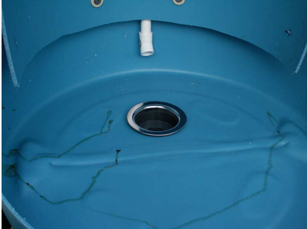
Detail of the sink drain and lower part of the 1/2" pipe
