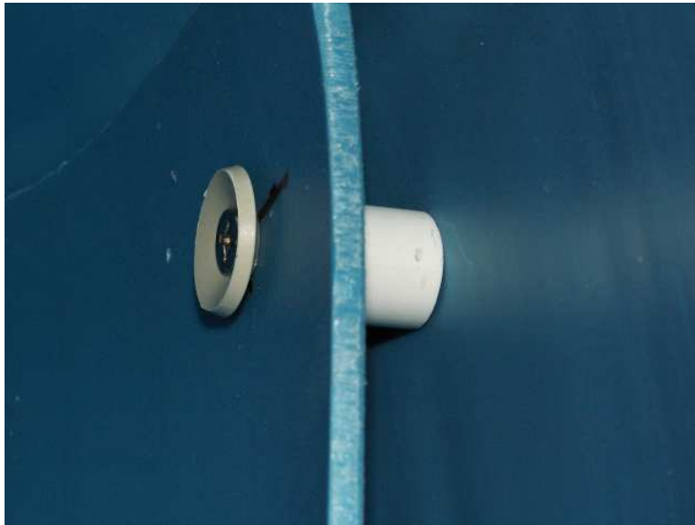
Detail of spacer to keep the false wall away from the back wall. It is a 1 inch long piece of the 1/2" PVC pipe.
